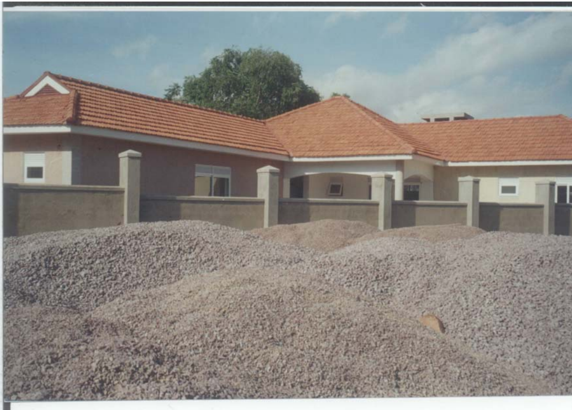
Side view of the House at Plot 37 Luzira and showing some of the materials (sand and stone aggregates) on site
