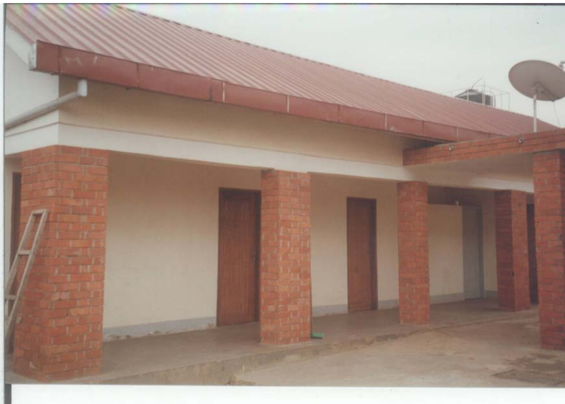
Servants Quarters for the house at Nyakabande Kisoro
