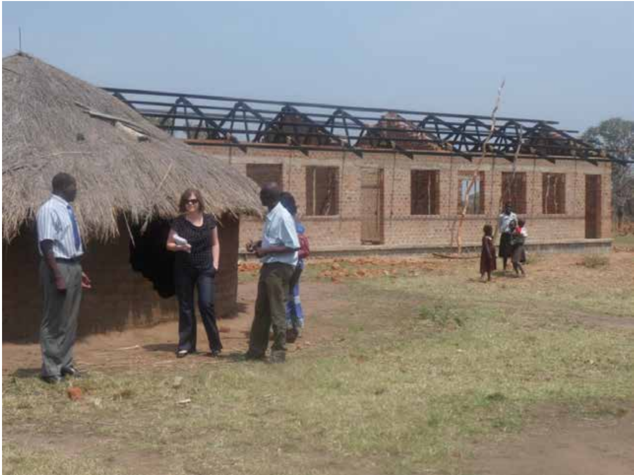
Monitoring school classroom construction sub project under NUSAF 2 Project
